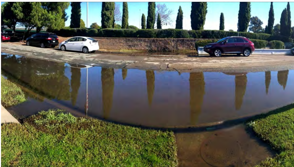
Figure 1.3 Veterans Court in the City of Alameda during King Tides. Groundwater intrusion into the sewer system provides a pathway for inland flooding when Bay tides are high. A high groundwater table and emergent groundwater flooding have caused pavement failures (May et al., 2023). (Photo credit: Kristina Hill)
