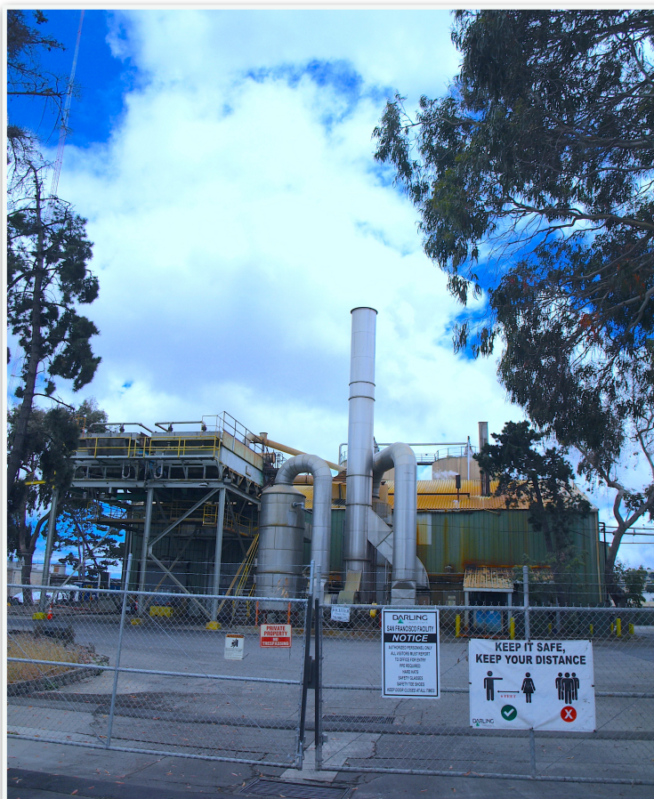
Figure 3. A portion of San Francisco Darling's rendering facility. Source: Photo taken by Elias Rodriguez.
