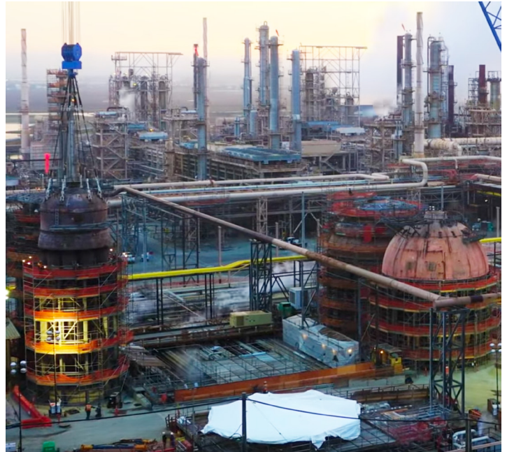
Chevron Richmond Refinery Fluid Catalytic Cracking Unit (FCCU) during major repairs
