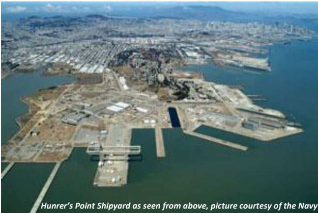
Hunter's Point Shipyard as seen from above, picture courtesy of the Navy
